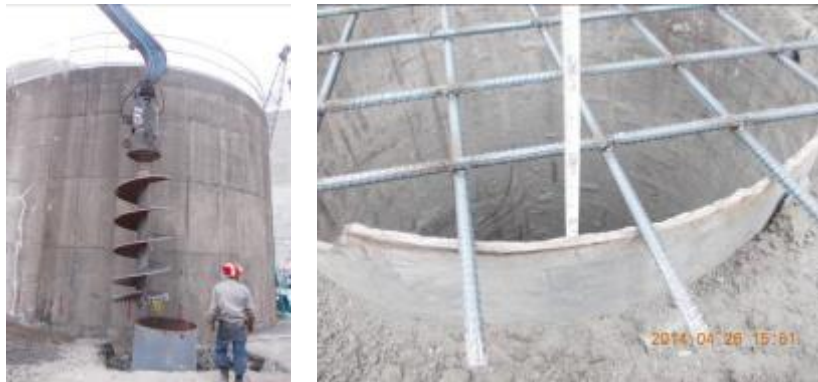
Pile Drilling
