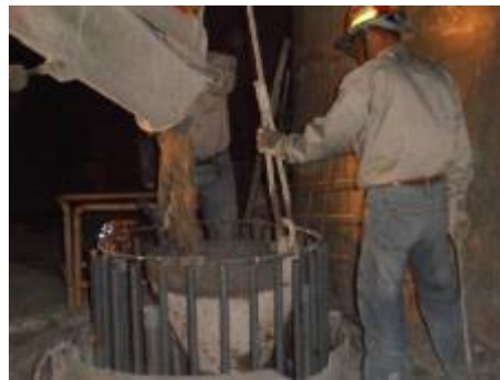
Concrete Placing
